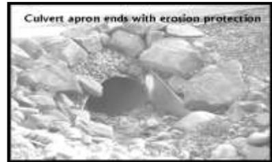
3. Erosion protection requires the placement of 6" to 12" diameter washed rock riprap to cover the pipe apron. The washed rock must match the community-approved standards. Improved driveway entrances four feet or less may be constructed as to enhance the property and comply with the specified and approved building materials for fencing and driveways. Please contact the ARC for specifications and approval.
